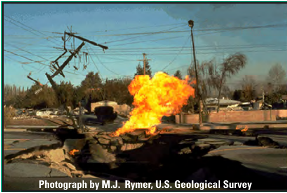
Natural gas pipeline broken as a result of the 1994 Northridge earthquake in southern California.
