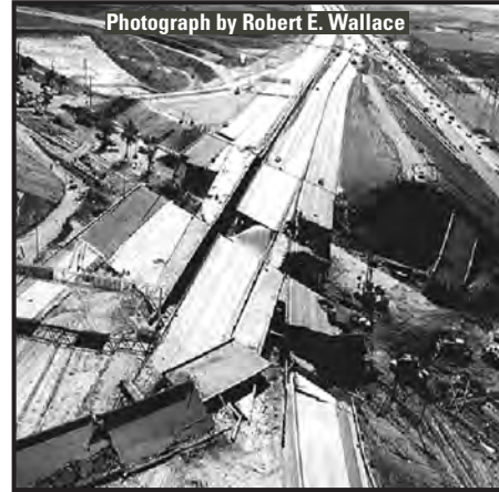
The San Fernando earthquake of 1971 collapsed freeway overpasses in southern California.
