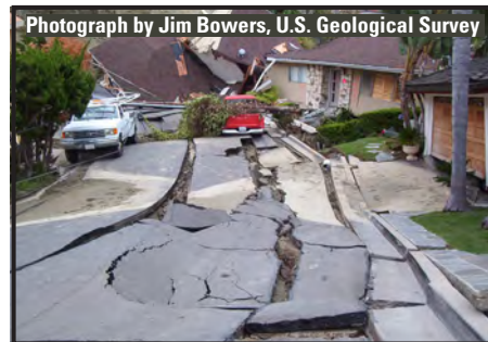
Landslide at Laguna Beach, California, June 2005. The landslide occurred after record heavy rainfall in southern California in the preceding months. It occurred next to the 1978 Bluebird Canyon landslide.
