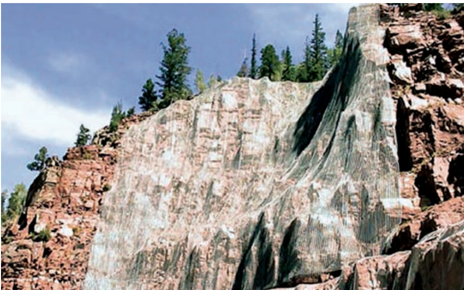
Figure C23. Example of a "rock curtain" that controls rockfalls in problem areas. (Photograph by Doug Hansen, High Angle Technologies, Inc.)
