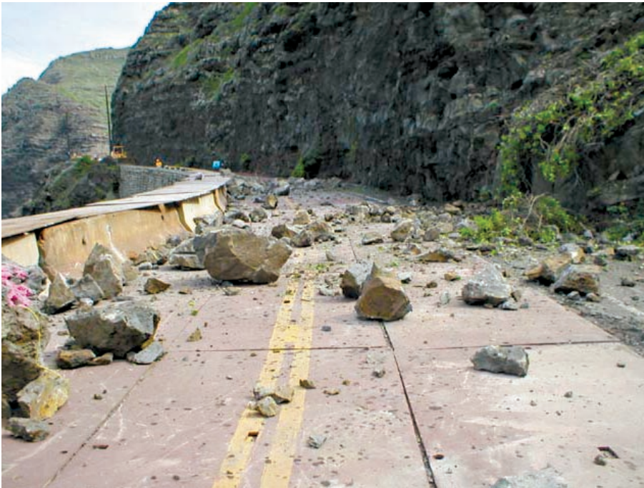
Figure C29. Rocks dislodged by scaling and blasting. (Photograph by Washington Department of Transportation, USA.)
