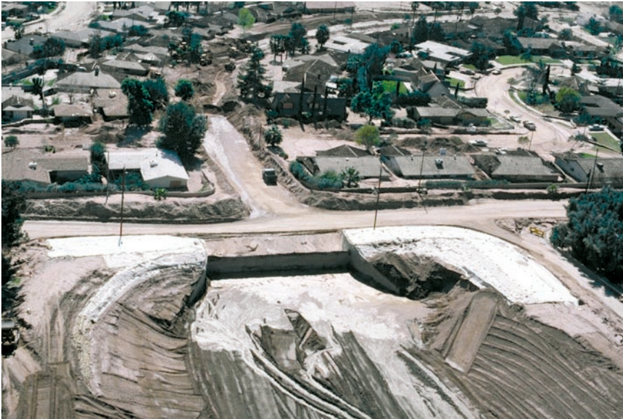
Figure C35. Aerial photograph of a debris-flow basin, constructed at the bottom of a slope in San Bernardino, California, USA. (Photograph by Doug Morton, U.S. Geological Survey.)
