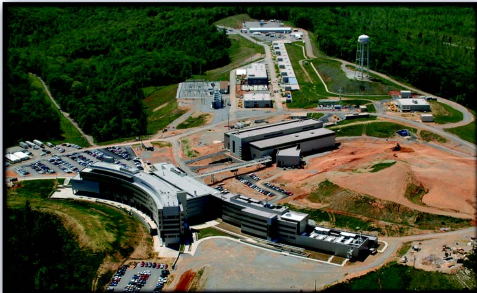
May 8, 2006, aerial view of the SNS site. Construction is complete except for a few finishing touches and landscaping.
