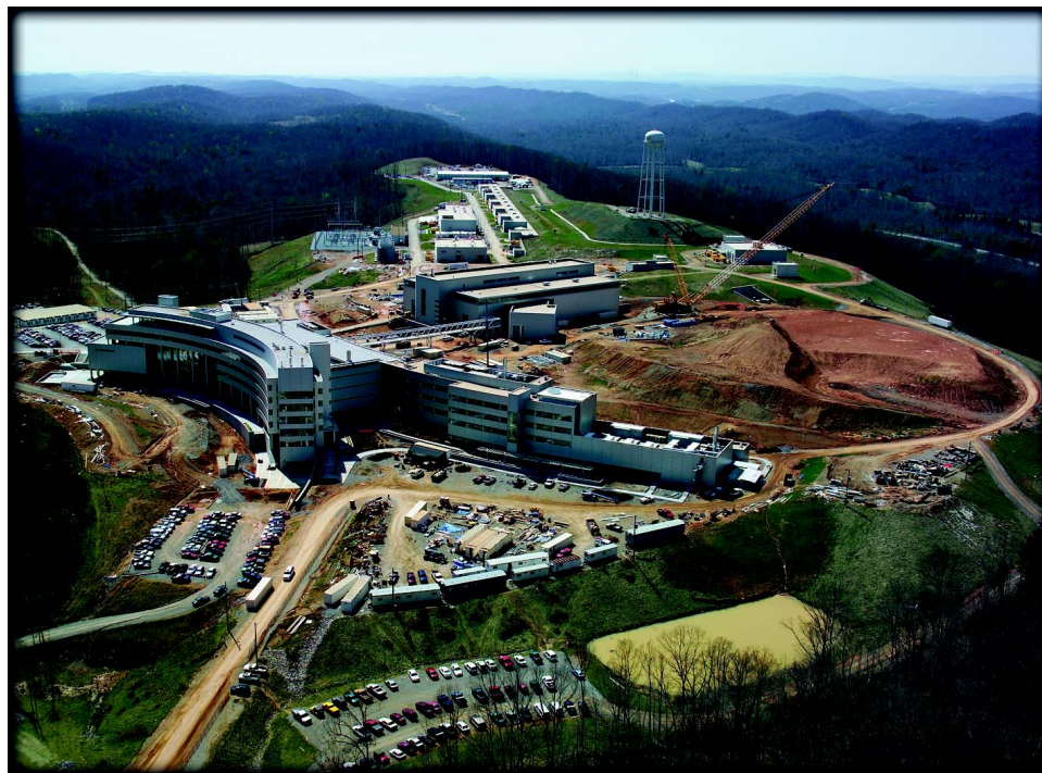
Westward view of the SNS site, April 2005. The CNMS is the curved building in the foreground that extends to the right of the SNS CLO. For more photos, see the SNS Photo Gallery at web.ornl.gov/sci/iris/search_sns.shtml .
