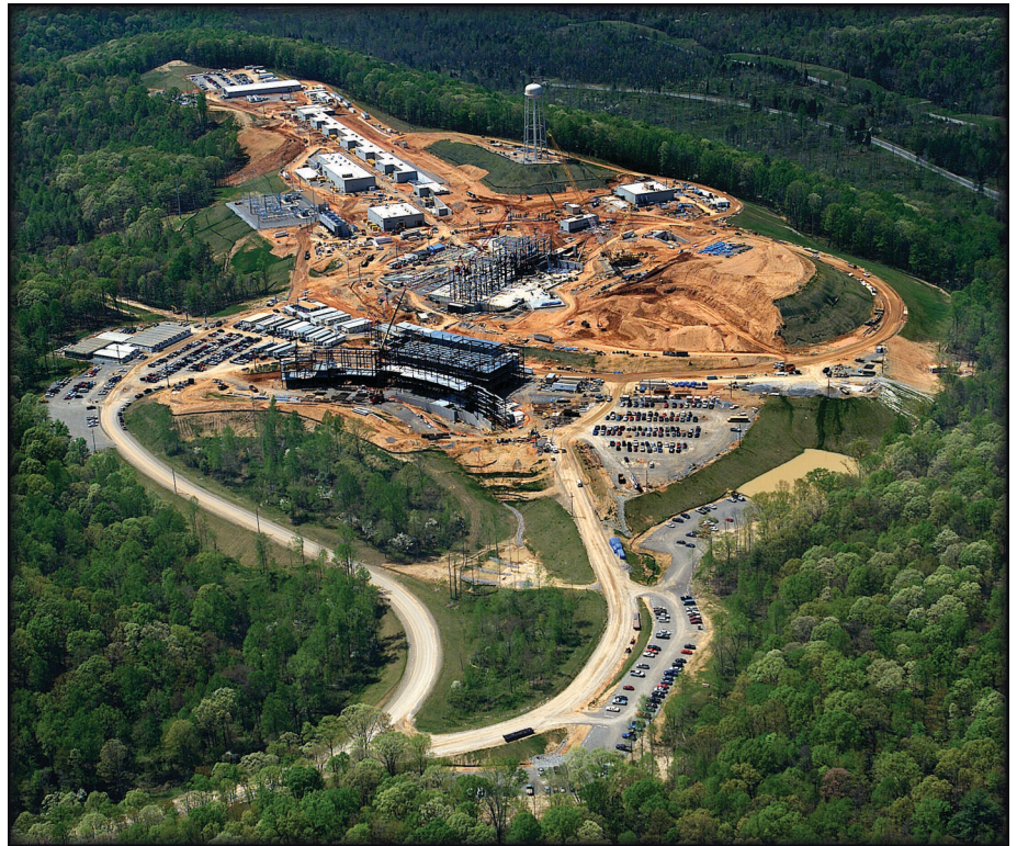
Aerial view of the SNS site, April 14, 2003.
