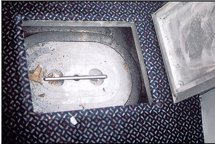
Figure 3-7 Access to “Main Deck” Manhole, Lightning
