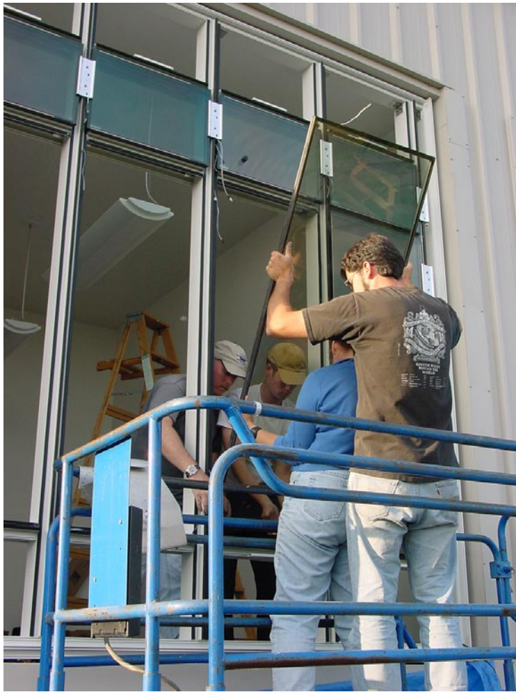
Figure 2. Installing windows
