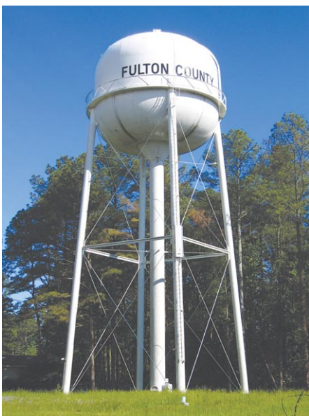
Public-supply water tank in Fulton County, Ga. Photograph by Alan M. Cressler, USGS.
