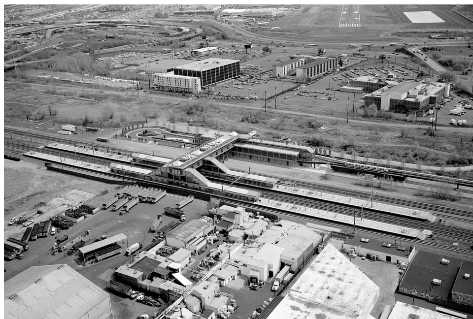
Figure 7: Train Station and Automated People Mover at Newark's Liberty International Airport
