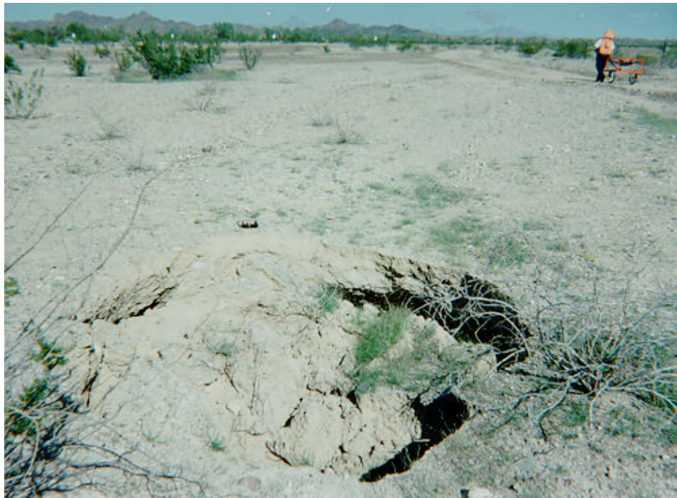
Unnatural subsidence features should be noted during the site visual inspection.
