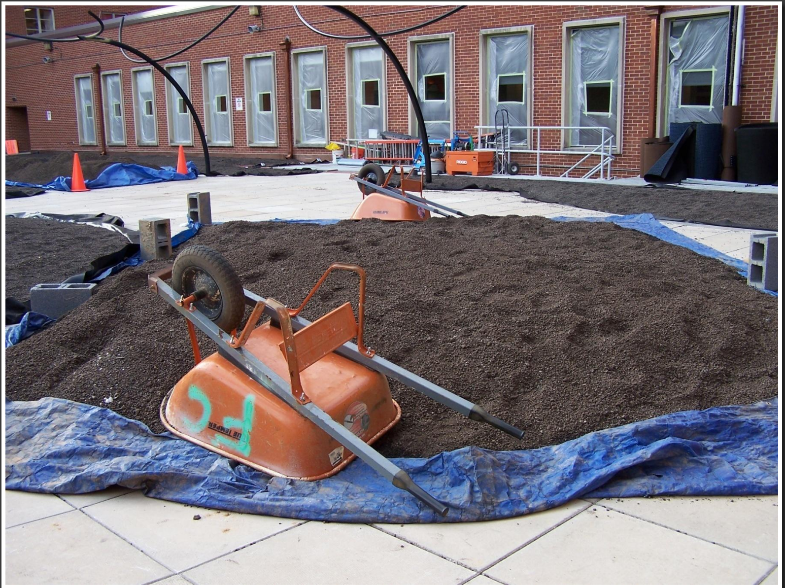
Enriched soil was then put on top of a weed barrier atop the fine rock.
