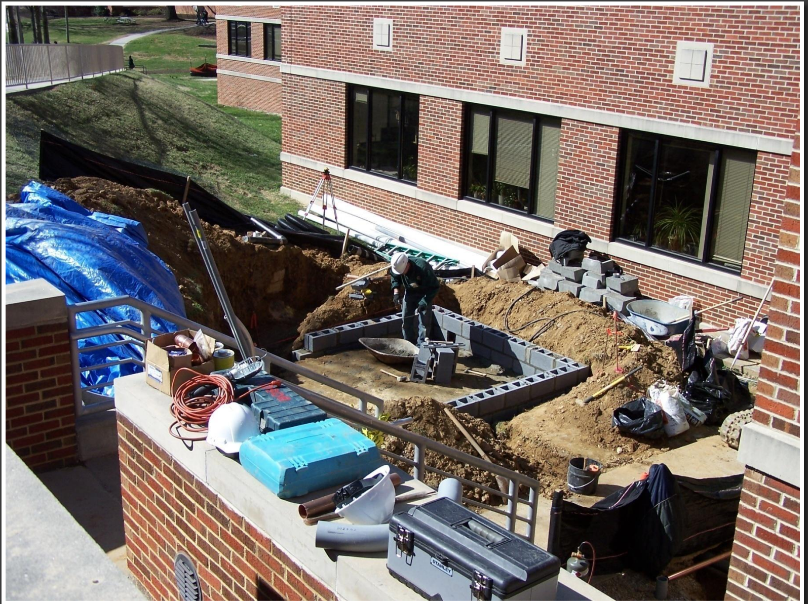
A concrete base was created for the 1500 gallon water cistern.
