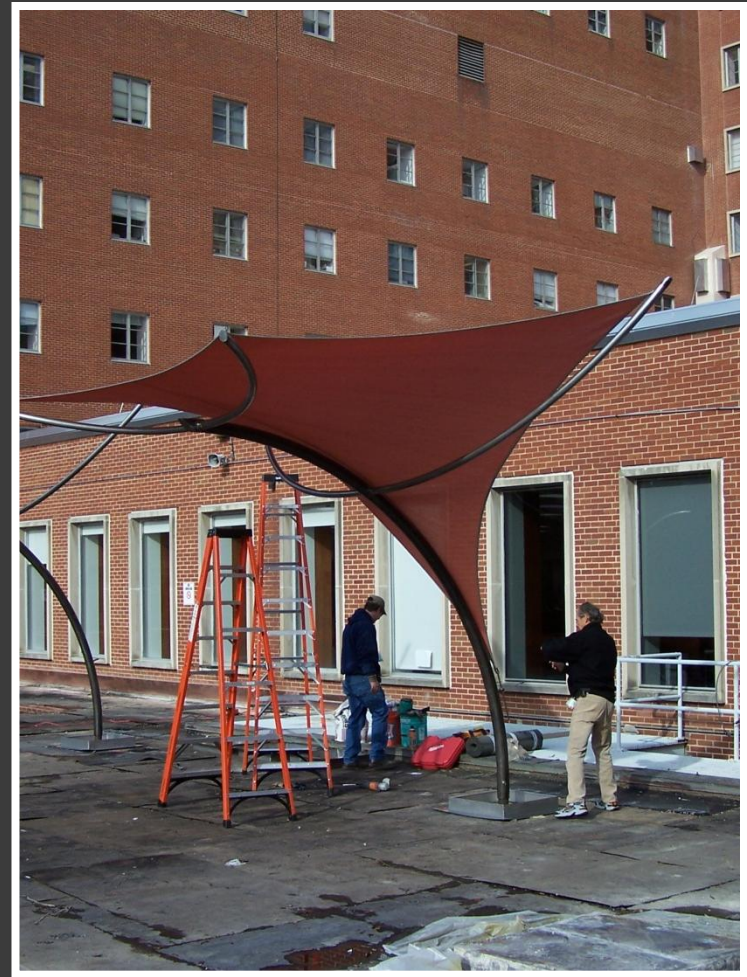
Then the canopy material was attached creating the Sunami shade structure.
