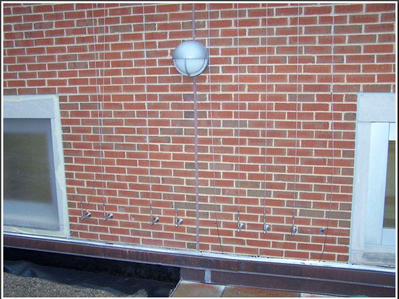
Aircraft grade cable was added to the wall that will allow vines to grow up the wall, further reducing the terrace heat levels.
