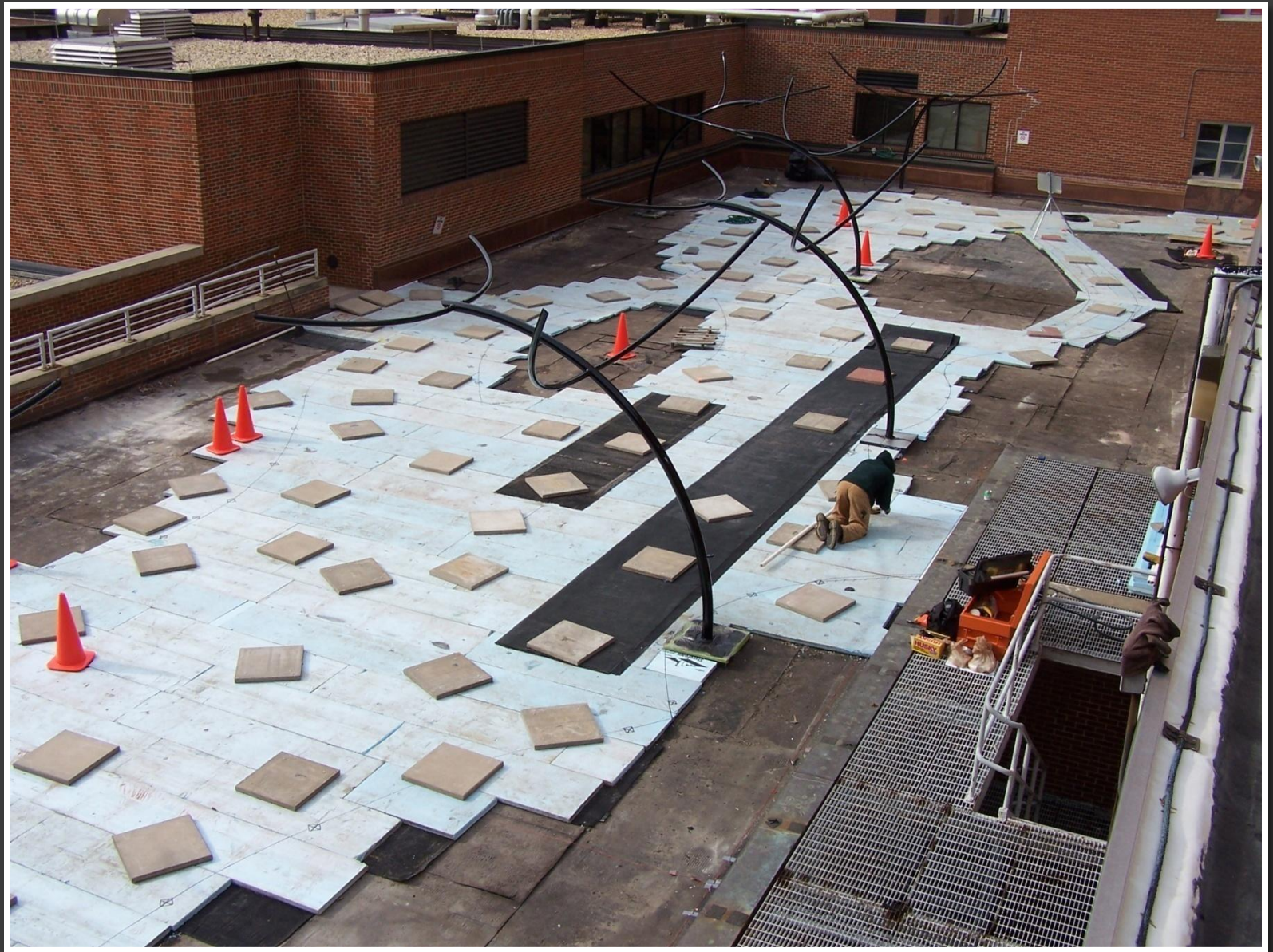
Foam insulation tiles were placed wherever the concrete tiles would go.
