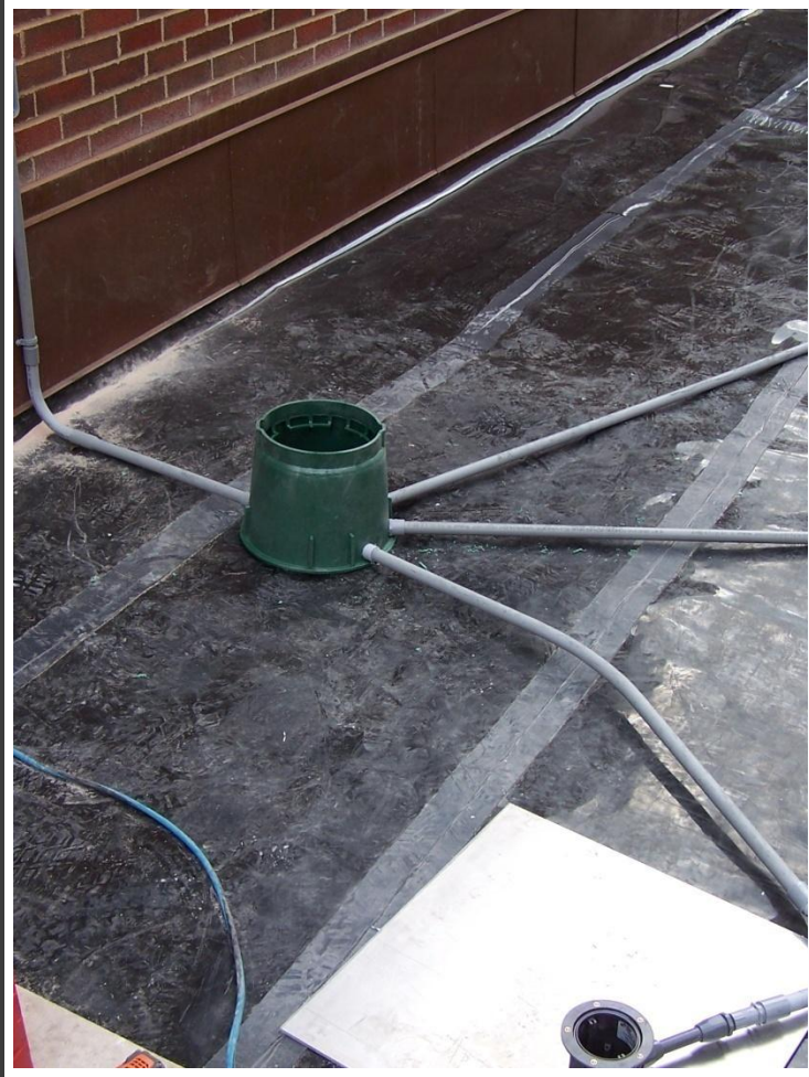
Electrical conduit and relay boxes were installed for light fixtures
