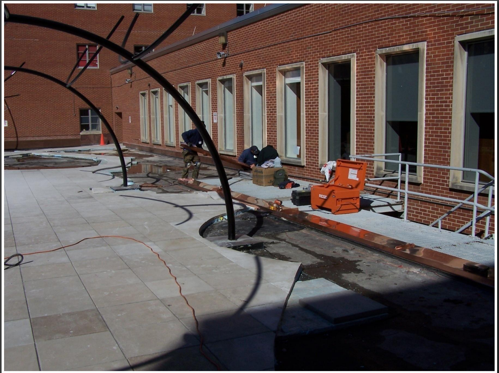
A beautiful copper cover was added to accent an existing stairwell.
