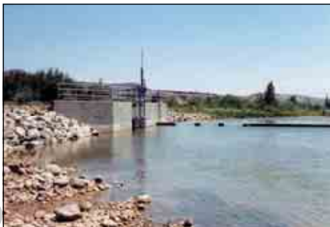
Rebuilt Pioneer Diversion on the lower Duchesne River
