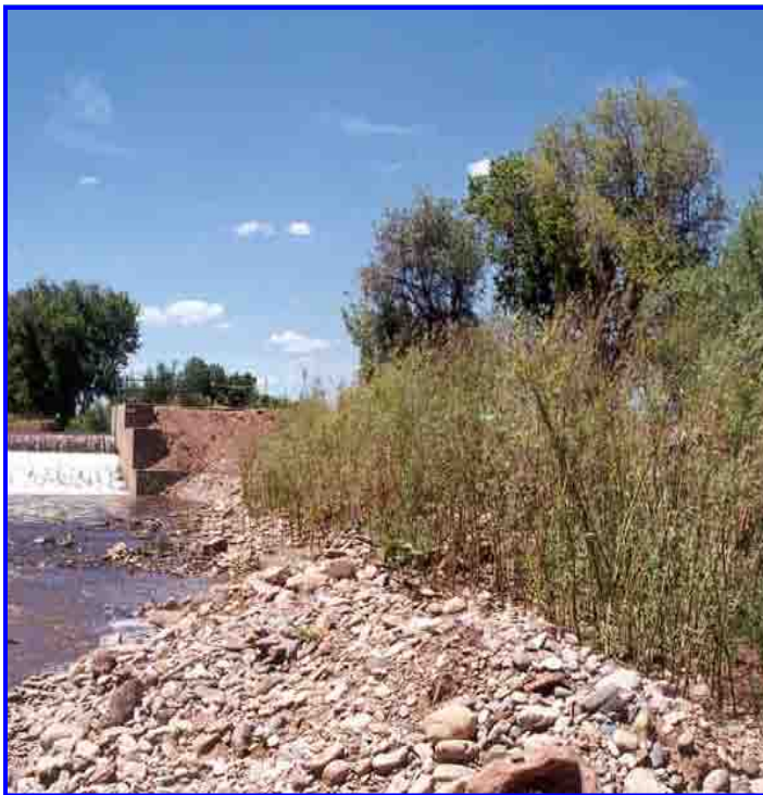
Before and after: Streambank stabilization is achieved by “deep planting” coyote willow whips; planting holes were augered in the rocky soil by using rotary hammers.
