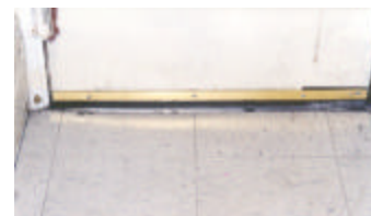
Install a doorsweep
