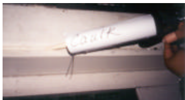
Caulk cracks and crevices
