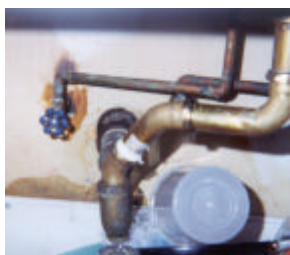
Repair water leaks
