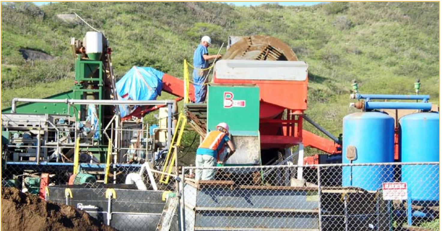
Soil washing treatment technology will be utilized at the small arms firing range restoration project at Camp Withycombe to clean the soil and reclaim lead for recycling.
