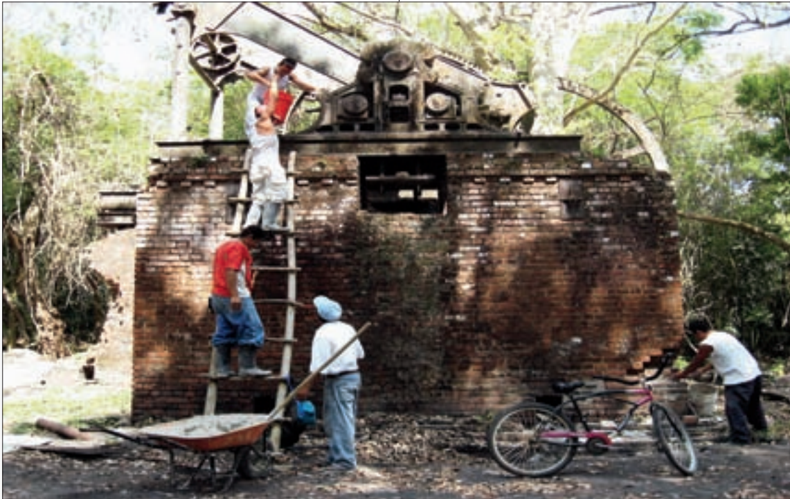
Restoration of the Dominica Old Mill Cultural Center U.S. Embassy Bridgetown
