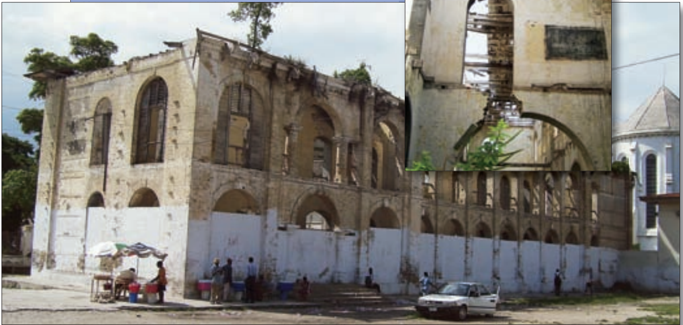
Grand Collège building before restoration U.S. Embassy Port-au-Prince
