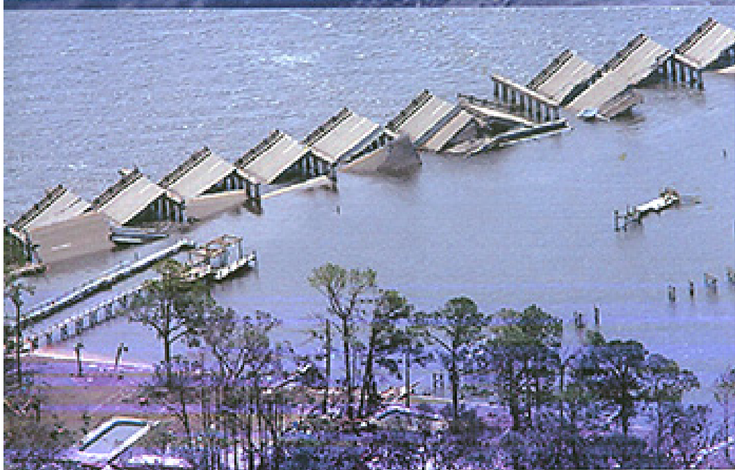
Figure 4.4 Hurricane Katrina damage to Highway 90 at Bay St. Louis, MS. (Source: NASA Remote Sensing Tutorial)
