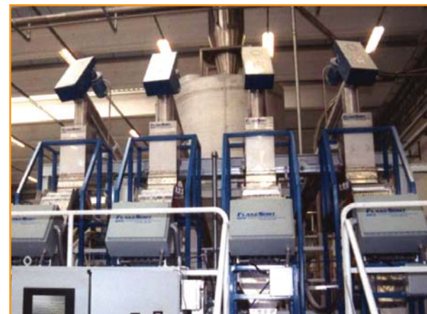
Second-generation FlakeSort™ unit installed in a recycling facility near Venice, Italy.
