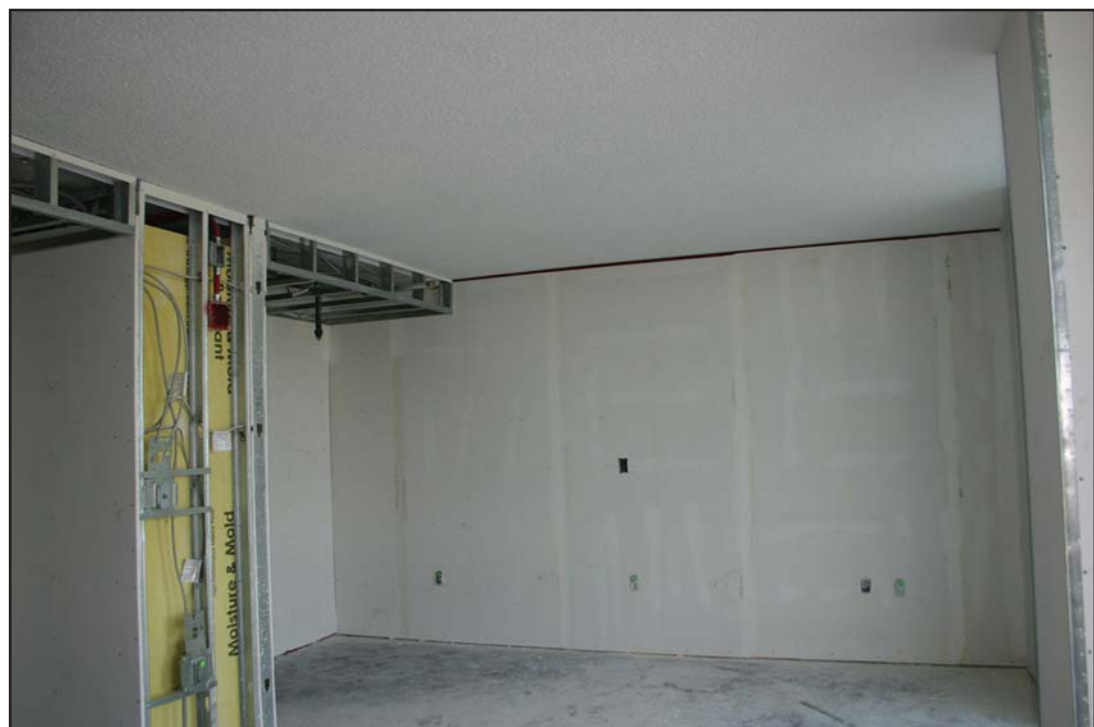
Finish work continues on residential rooms.
