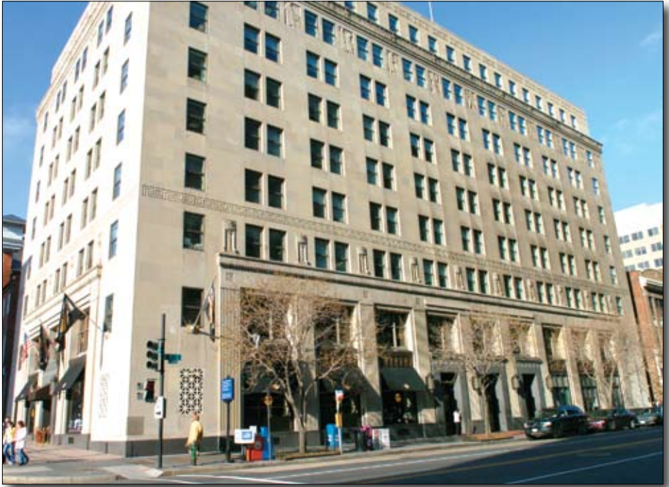
FEC Building in downtown Washington, D.C.
