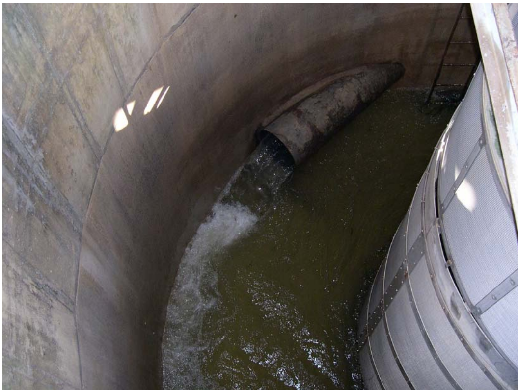
FIGURE 2.—Top and inside view of the recessed holding tank, TFCF, California.
