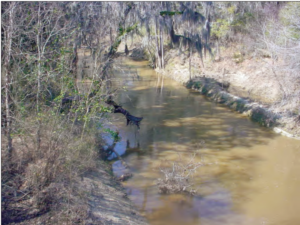
Figure A20. Downstream of Seaboard Coast Line Railroad bridge, Montgomery, Alabama. (See figure 7 for location.)
