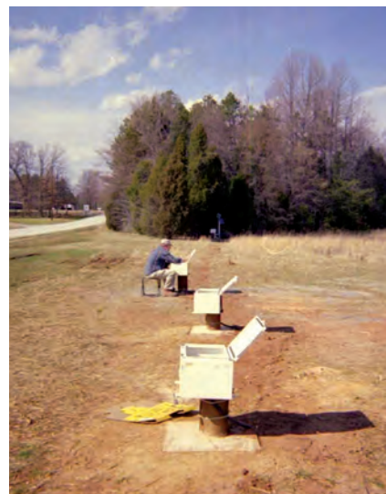
Ground-water-level monitoring equipment being installed at well cluster MW-2 (photograph by Stephen Howe, retired, U.S. Geological Survey).
