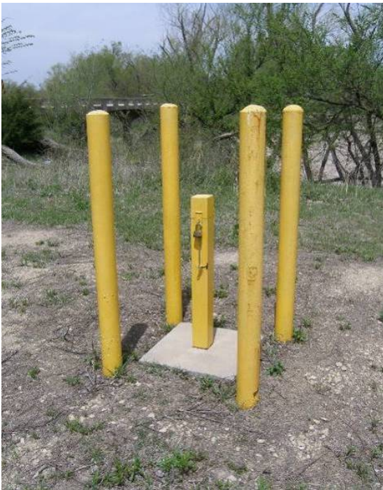
Figure 1-3: Monitoring Well near the River
