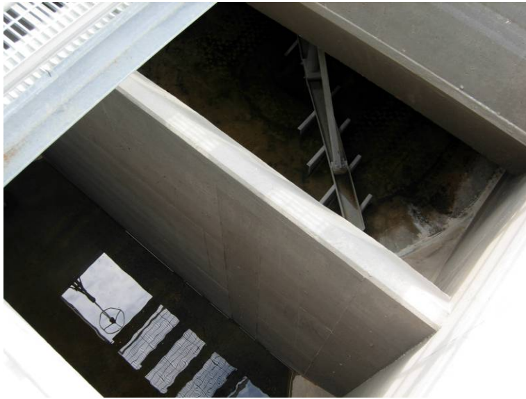
Tank used to remove solids from the water
