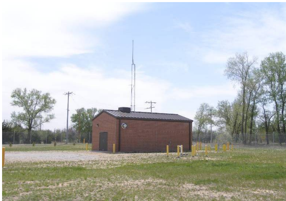
Figure 2-2: Recharge Recovery Well Site with SCADA Tower
