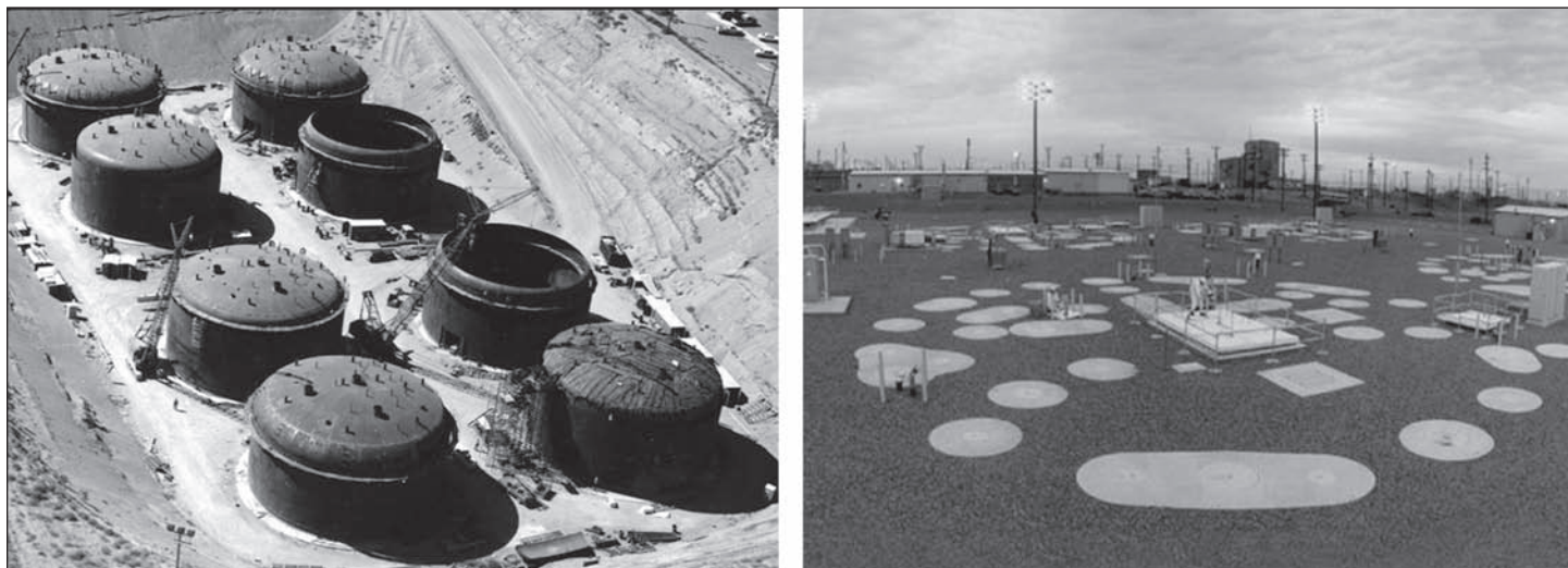
Figure 1: Double-Shell Waste Tanks under Construction and Completed Tank Farm at DOE's Hanford Site
