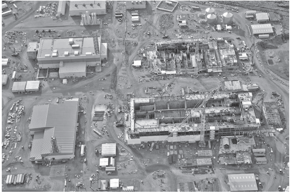
Figure 2: Waste Treatment Plant Primary Facilities under Construction as of November 2008
