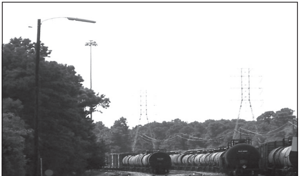
Figure 5: Light Towers at a Rail Yard in Houston
