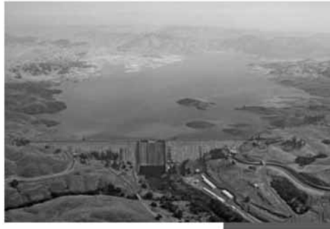
Friant Dam, on the San Joaquin River, California. Temperance Flat Dam would be a new structure constructed on the San Joaquin River, above Friant Dam, which would provide much needed water supplies and hydroelectric power. Source: USBR
