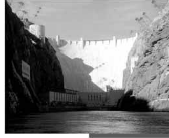
Hoover Dam, on the Colorado River. Source: USBR.
