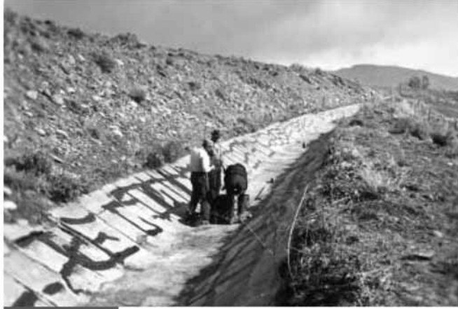
Opportunities exist to improve water conservation in Western agriculture, such as finding ways to minimize channel seepage losses. However, conservation alone cannot supply enough water for the tens of millions of new residents moving to the West. Source: USBR.
