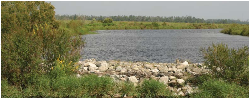
On the Barataria Basin Landbridge, rock dikes slow erosion along bayou shorelines, preventing archaeological sites and hunting and fishing camps from washing away. Project planners worked with property owners and users to ensure the dikes didn't block access to the wetland.
