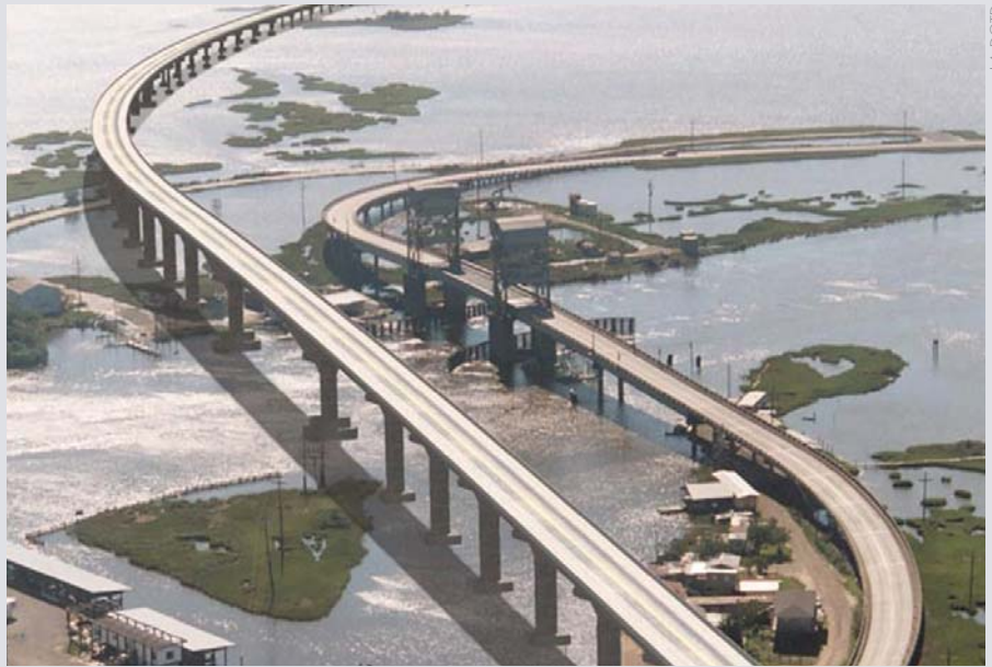
A March 2007 groundbreaking launched Phase 1A of improvements to LA Hwy 1; a new fixed-level Leeville Bridge. Shown in this artist's rendering, the new bridge will soar 73 feet above Bayou Lafourche and Boudreaux Canal.
