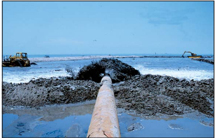
On East Timbalier Island, sediment is being pumped onto the marsh platform.
