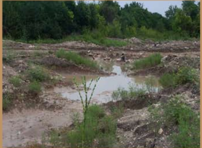
Tank Trail Low Water Crossing Project - Before
