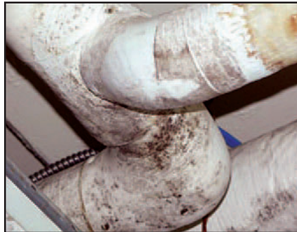
Figure 4: Leaking Pipes Caused Mold and Mildew Damage at Naval Amphibious Base Little Creek
