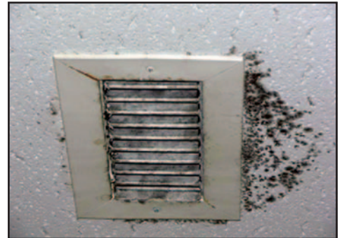
Figure 4: Leaking Pipes Caused Mold and Mildew Damage at Naval Amphibious Base Little Creek
