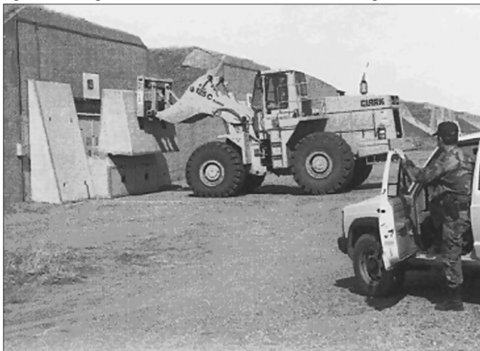
Figure 1: Adding Concrete Barriers That Secure an NNSA Storage Vault
