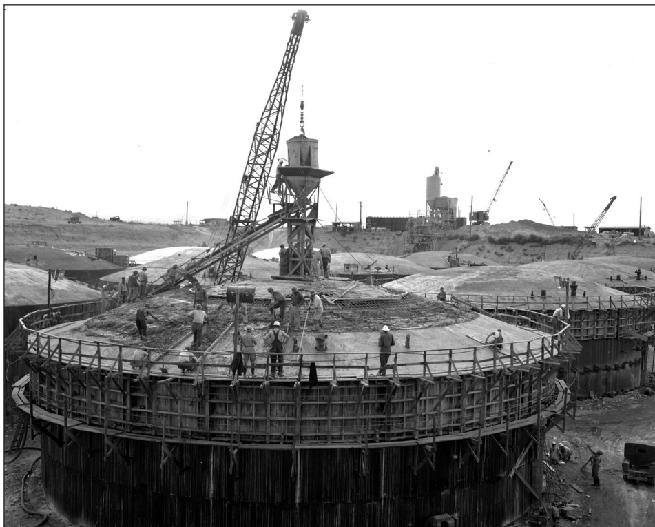
Figure 2: Waste Storage Tank Under Construction at DOE's Hanford Site, September 1947
