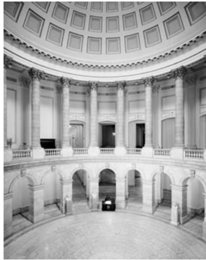
The Cannon House Office Building Rotunda
