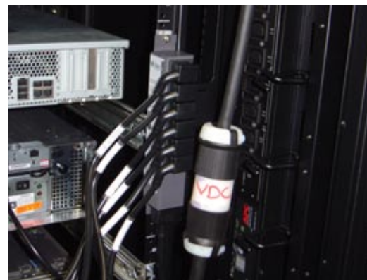
Figure 4. DC connectors need to be standardized similar to AC connectors.
