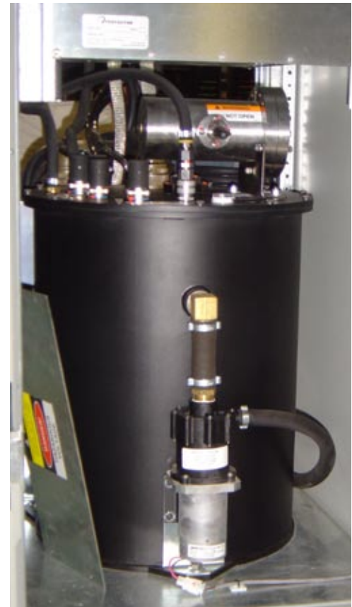
Figure 1. Flywheel uninterruptible power supply (UPS)
