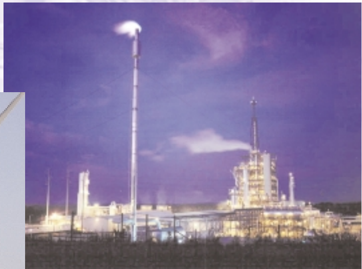
The Washbush River Coal Gasification Repowering Project, an Integrated Gasification Combined Cycle (IGCC) facility, is considered one of the cleanest coal-based power generation facilities in the world. It is owned by General Energy and Cinergy.
