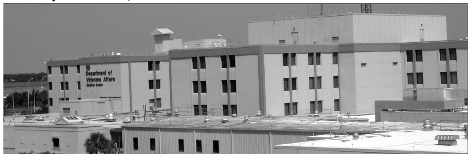
VA Facility in Charleston, South Carolina
