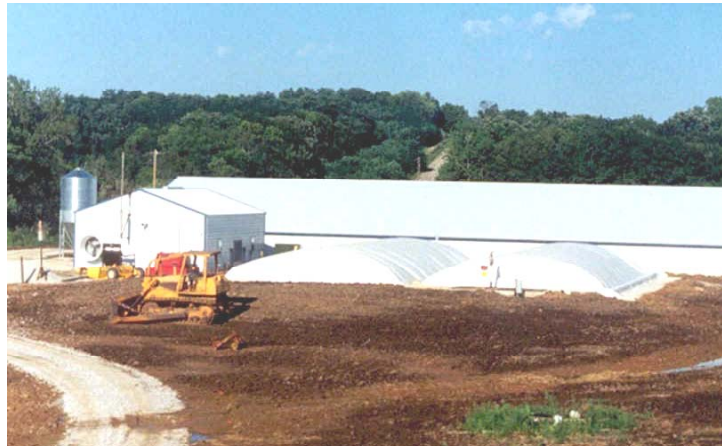
Construction of a complete mix anaerobic digestion system
