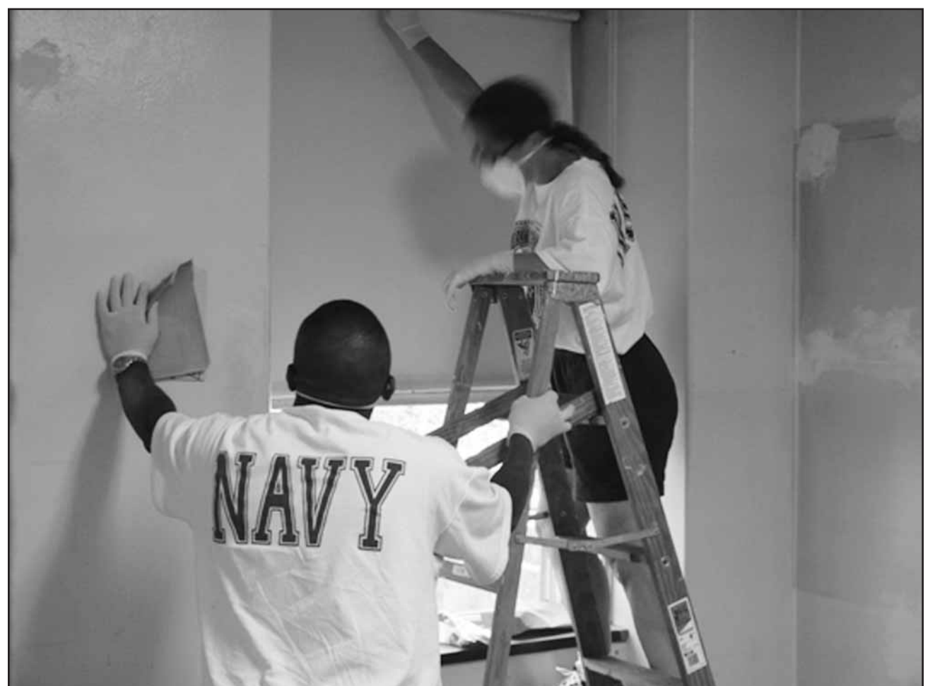
Two chief selectees paint the new Information and Referral Room.
