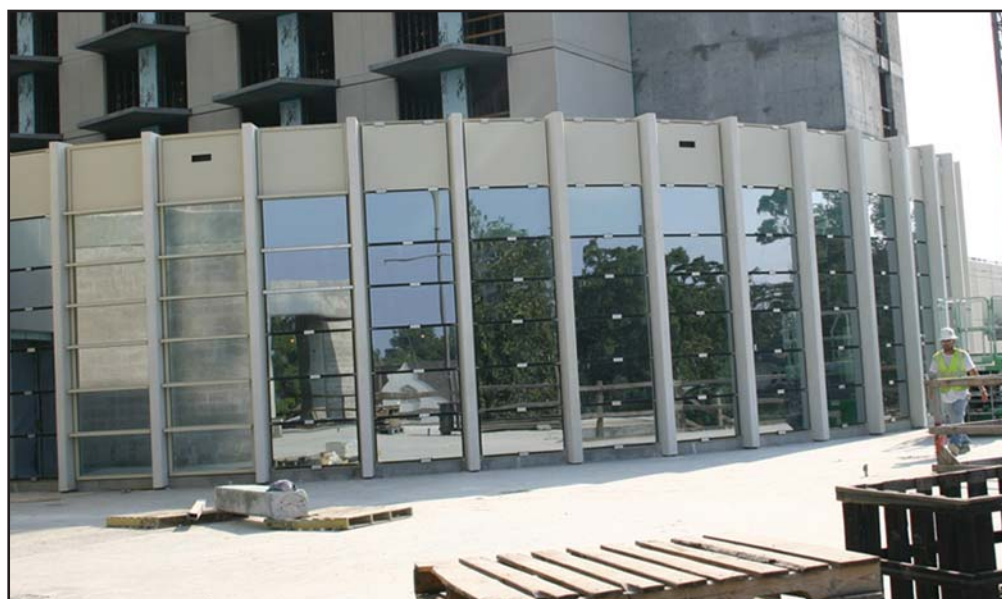
The dining room and outside dining area, located at the front of the building, between Towers B and C.
