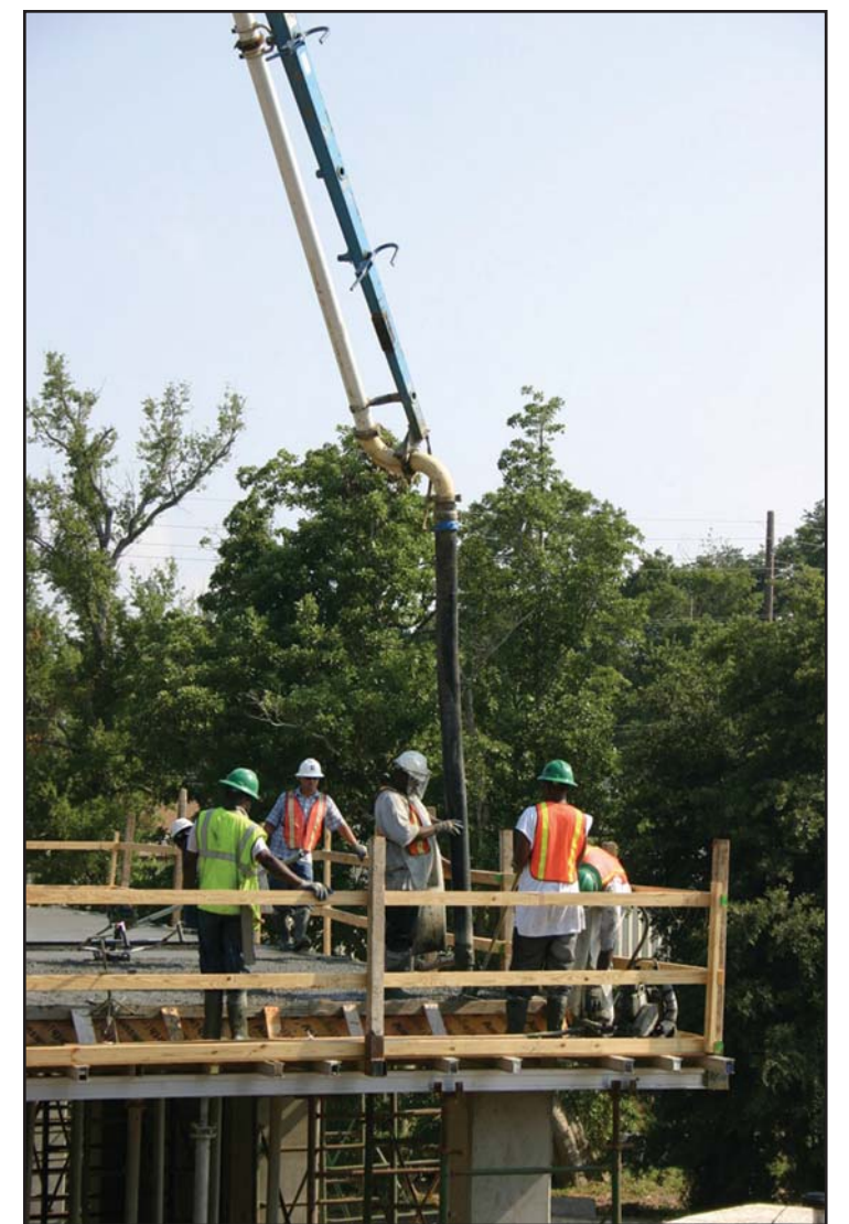
Concrete placement on the generator pad behind the main building.
