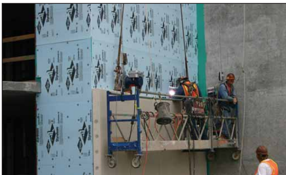
Pre-cast concrete panels being installed on the south end of Pavilion B.
