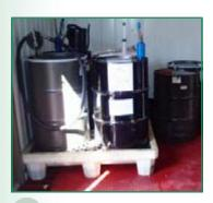
HAZMAT is stored indoors with secondary containment preventing storm water pollution
