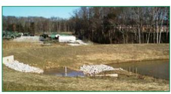
Storm water gets further treatment in an extended detention pond prior to discharge to the stream
