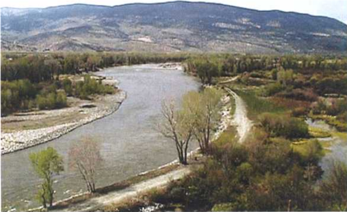
Bank stabilization using rip-rap along the Yellowstone River.
