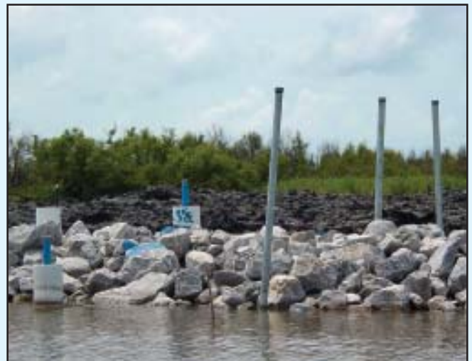
Typical view of geotechnical instruments (USACE).
