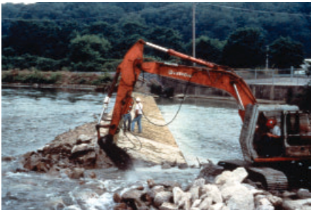
Left: Breaching dam
