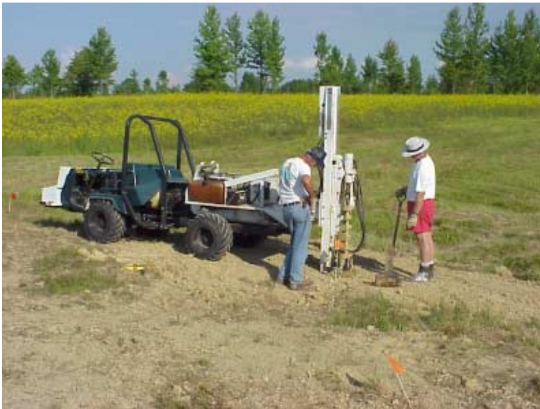
Figure N-3. Vertical drilling by Simco Earthprobe 200.
