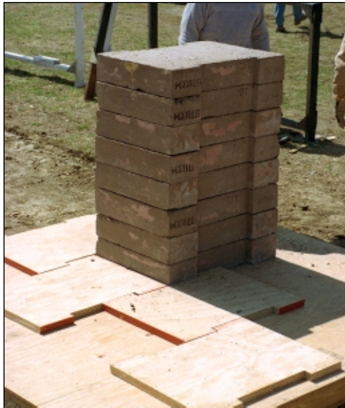
Figure 4-8. SACON wall construction using spacers.
