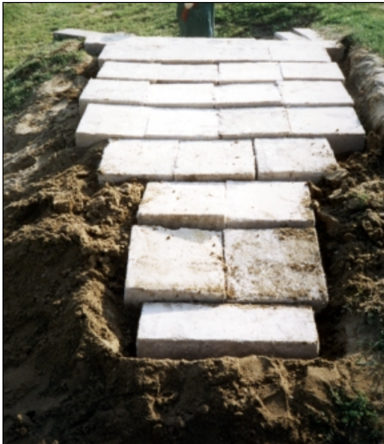
Figure 4-21. Berm (soil cover not installed), Fraser Range.
