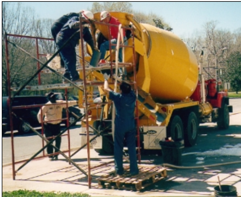
Figure 4-4. Mixing SACON.
