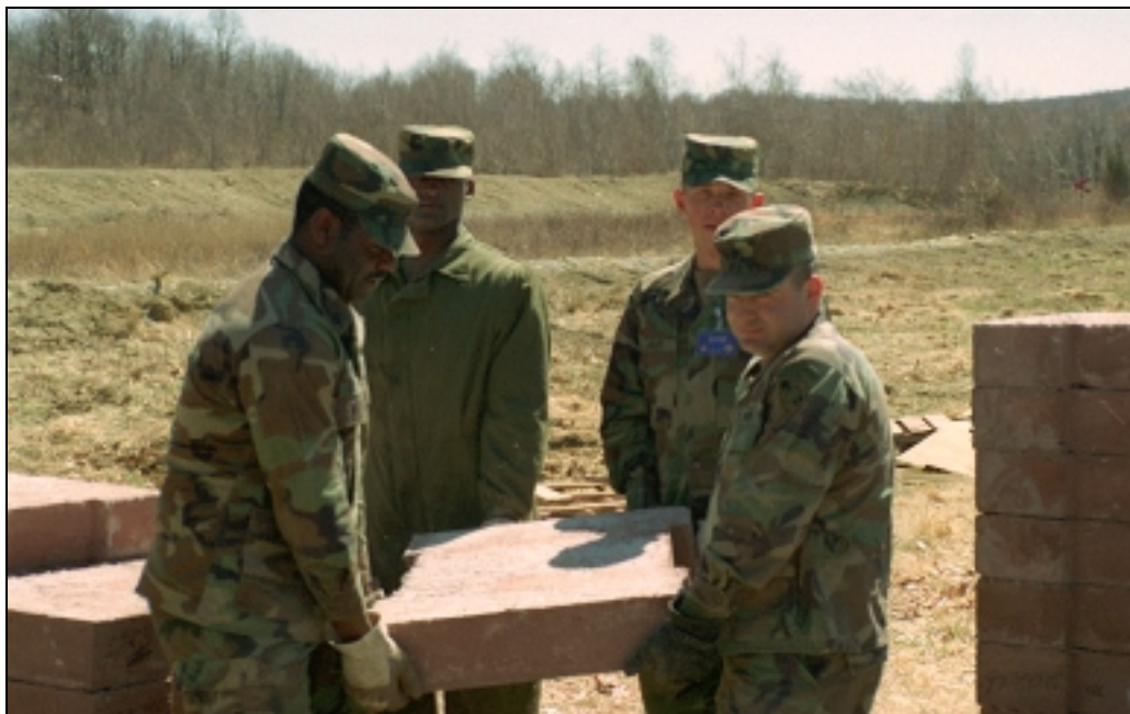
Figure 5-17. Four-man lift - 200-pound SACON block.
