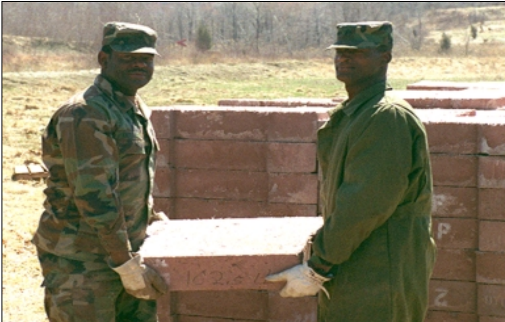
Figure 5-18. Two-man lift - 100-pound SACON block.
