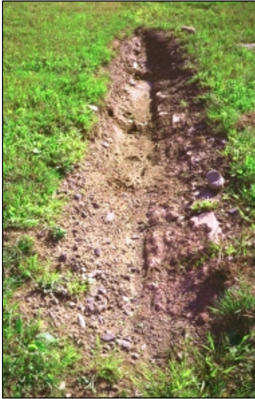
Figure 5-5. Typical erosion trough before SACON installation.
