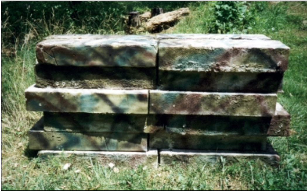
Figure 4-17. SACON backstop (block wall, Ditto Range, 50-meter right target, 26 June 1997).
