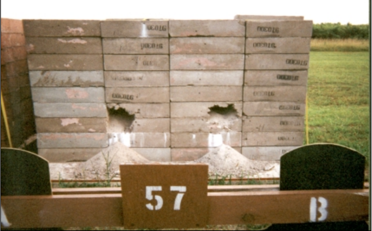
Figure 4-42. Typical cavity, Fort Knox Canby Hill Range.
