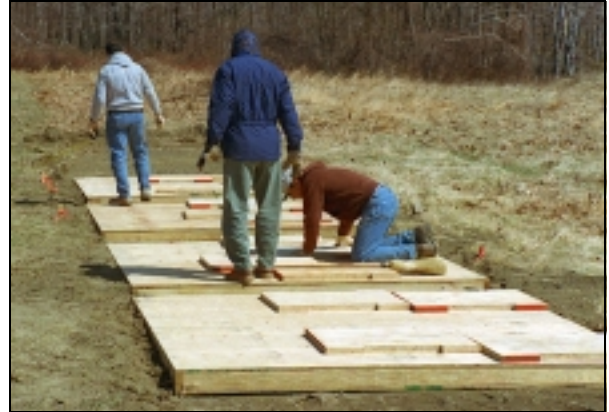
Figure 4-7. Plywood base for walls.
