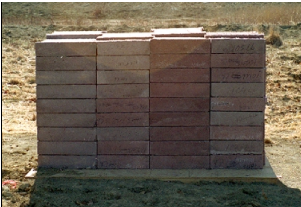
Figure 4-9. SACON wall on USMA West Point 25-Meter Range.
