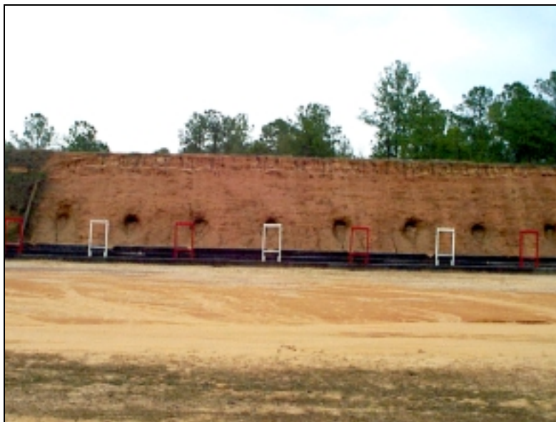
Figure 5-50. Soil berm bullet trap.
