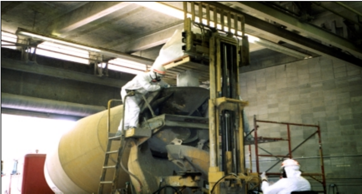
Figure 4-38. Mixing in recycled aggregate.
