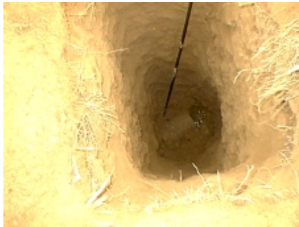
Typical excavation at JPG IV
