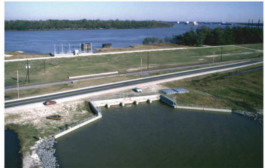
Caernarvon's five box culverts.
