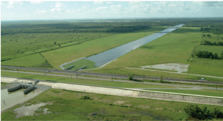
Davis Pond Freshwater Diversion Structure
