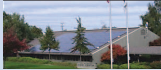
Solar units on the Ashland Police Station.
