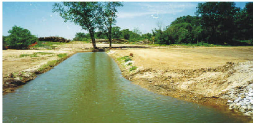
View looking west of the permanent storm water drainage channel.
