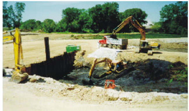
Typical sediment removal operations from the Unnamed Tributary. Swamphoe (seen in sediment bed) excavates sediment and transfers it to the edge of the bank. Trackhoe removes the transferred sediment and loads it directly into off-road hauler to be transported to the stabilization pond.
